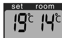
G: The required temperature on the left, the measured temperature on the right.
